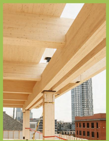
Glulam columns and beams supporting CLT roof panels
