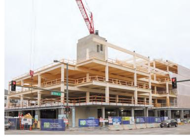
Mass timber reduced construction time by 20%
