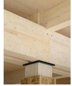
Column connected to CLT beam and girder
