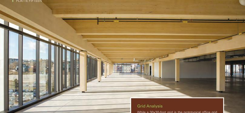
Kingsley added, "If we'd used the topping slab as the diaphragm, it would have limited future tenant improvement options. Using the CLT frees the topping for possible modification without shear transfer issues down the road, giving future tenants more flexibility."
